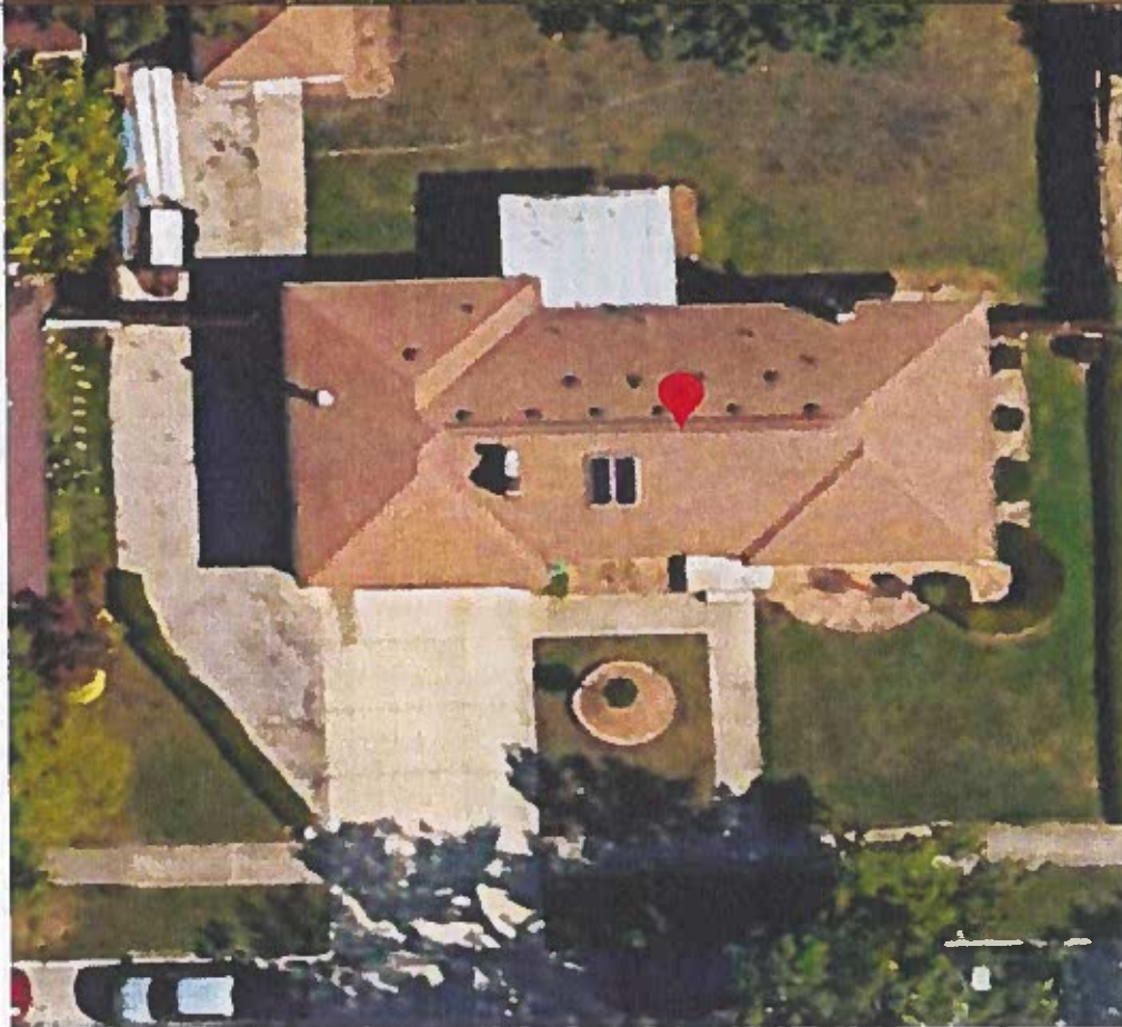
13672 Argyle St (Access Drive) Gravel) No Permit (last visit was 2018)
