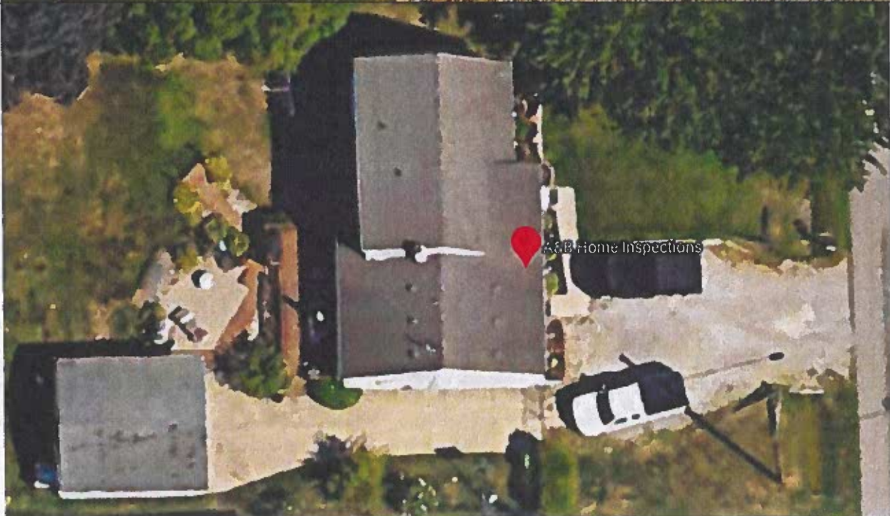
15300 Drysdale St (Access Drive) (Gravel) No Permit (last visit was NA)
