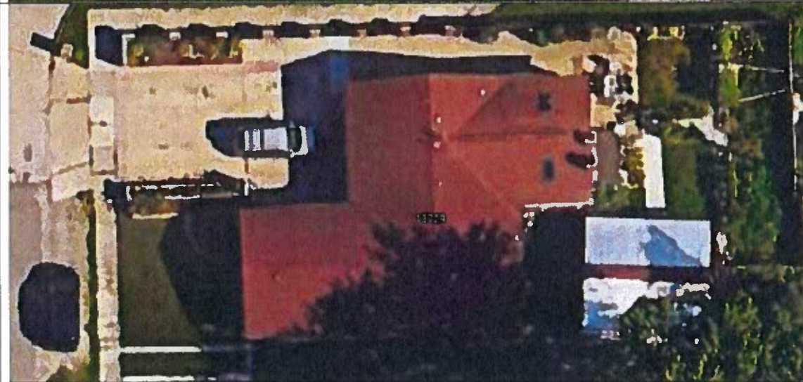
13729 Humphrey St (Access Drive) No Permit (last view NA)
